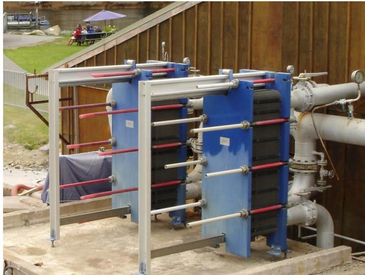
**Figure 3.2.** Plate heat exchanger at the Taupo Prawn farm (Thain et al 2006)
