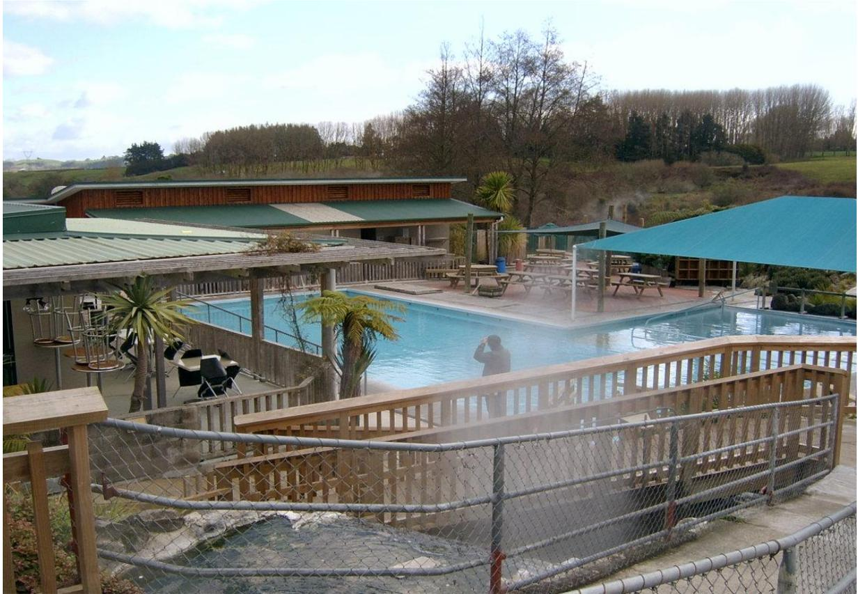
Photograph 1: Geothermally supplied swimming pools at Waikite, Waikato region. An open channel for heat loss can be seen in the foreground.
