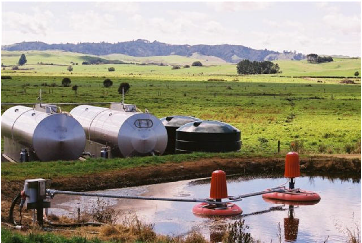
Figure 8. Two of Three ISE Digesters Producing Bacteria-Free Fertiliser and Methane Gas at Orni Downs Dairy Farm [ISE-2004, NZDE-4-2004].
