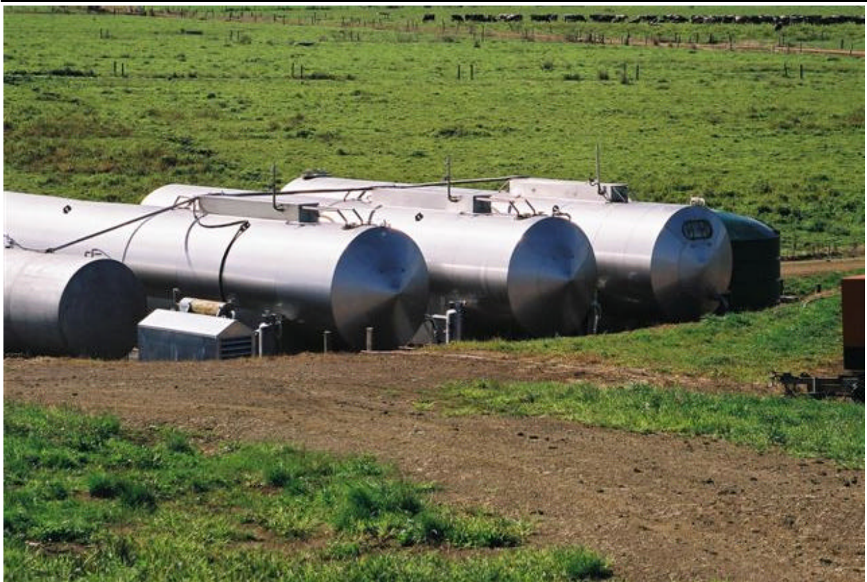
Figure 4. Three ISE Digesters Producing Bacteria-Free Fertiliser and Biogas for a 53 kVA Generator (running for 7 hours/day) [ISE-2004].
